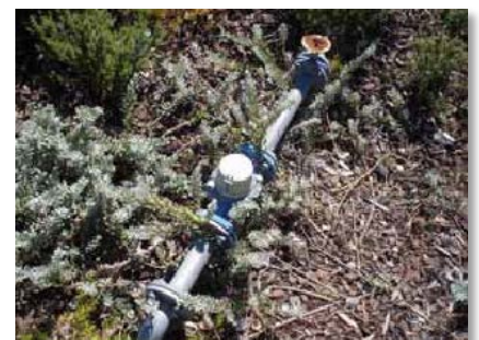
Image courtesy of the Water Corporation
