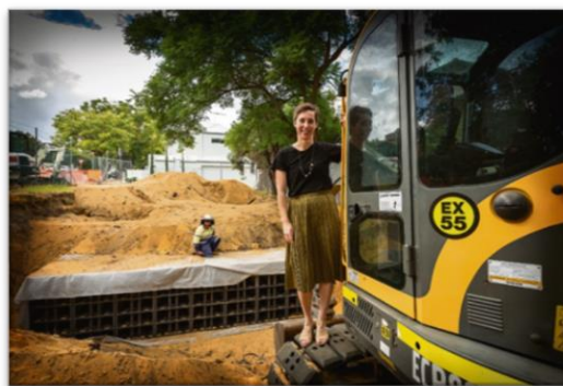
Over 300 stormwater cells were installed
