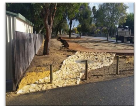
Bubble-up pit & overland flow path
