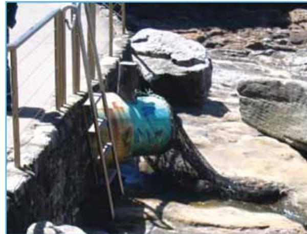
Release nets – netting installed on pipe outlets to collect litter
